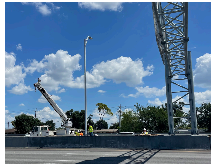
Light pole installation at Ramp G
