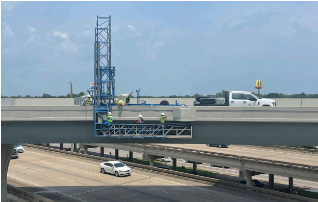
Conduit installation, I-10 Loyola Interchange
